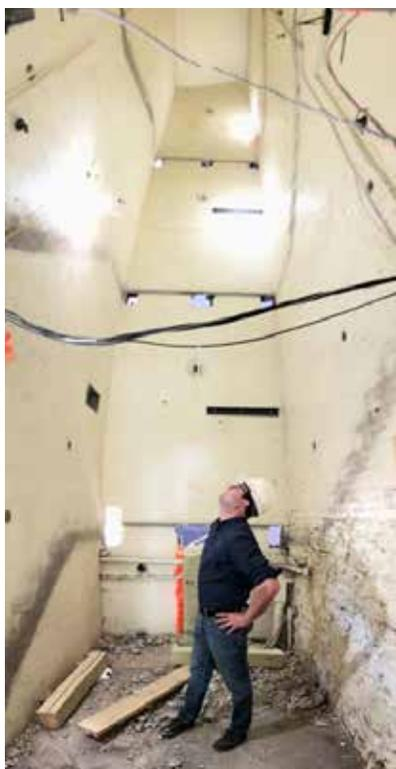
*April 30, 2020: the old back stairs removed to make way for the elevator*
