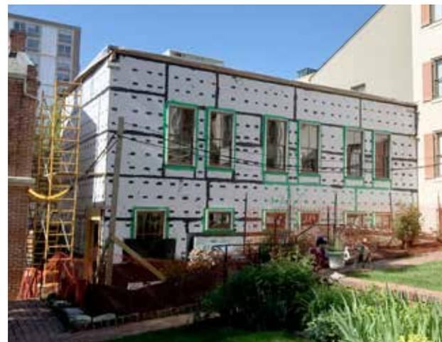
May 1, 2020: Windows installed making the facade ready for brickwork
